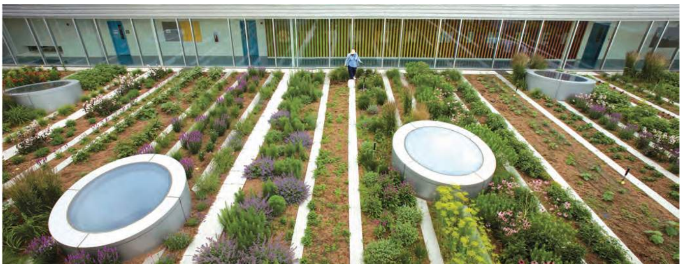
Fig. 24 Garden plots are divided by linear strips of recycled plastic. Photo by Scott Shigley.
