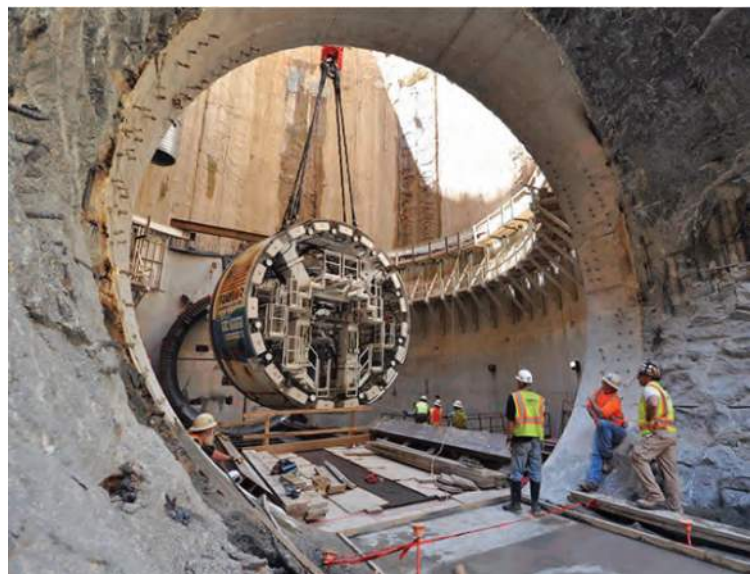
Fig. 4 Charismatic boring machine used to dig tunnel below Anacostia River. Image courtesy of DC Water.
